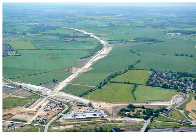
Figure 20: Aerial photograph of the A5-M1 road corridor, looking east from Watling Street
