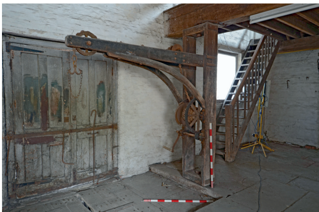
Figure 10: The Anchor Brewery, showing a hoist in the ground floor loading bay
